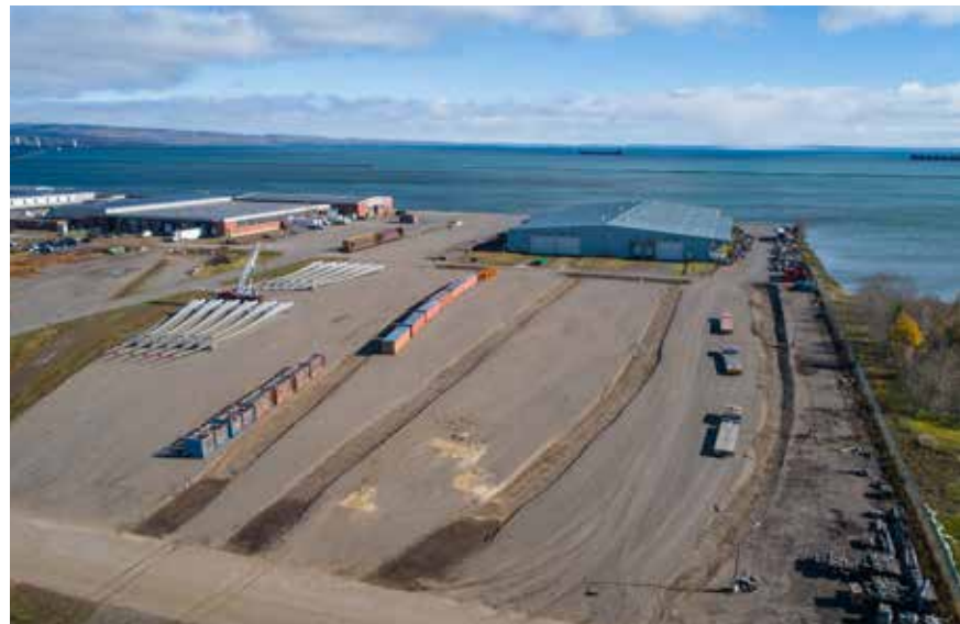
New laydown pads, constructed in 2018 as part of the terminal reconfiguration, were being used for cargo staging in September 2018
